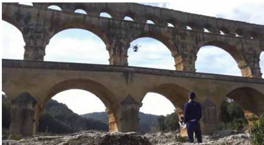
A low-altitude flying drone captured thousands of millimeter-resolution images of the Aqueduc de Roquefavour Roman aqueduct in Ventabren, France.
